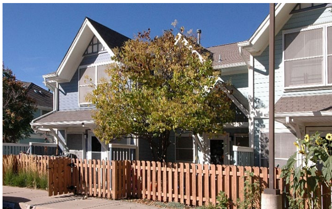
Existing Building at Woodlands
