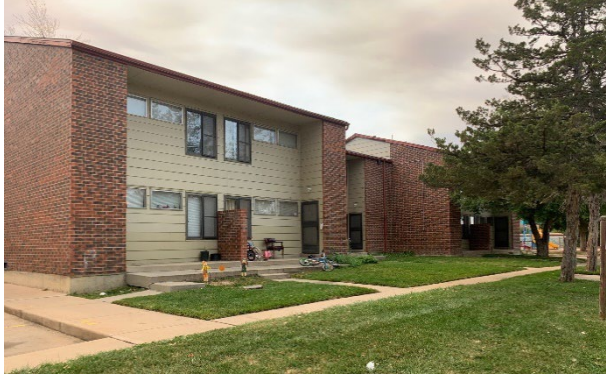
Existing Building at Madison
